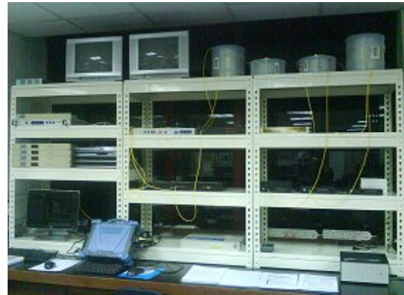
Figure 4. Testing on FTTH network system
